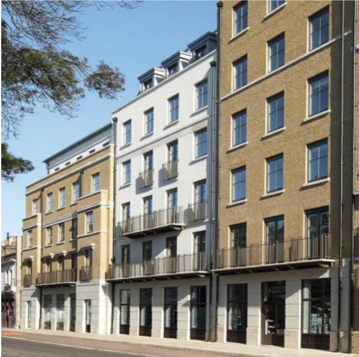
Figure 21: Taller ground floor windows, symmetrical glazing that is well proportioned and taller on the ground floor than at upper levels.
