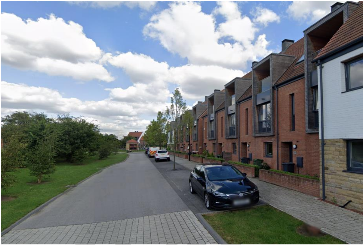
Figure 18.1 and 18.2 images showing i) a place with frequent doors and windows facing a street and ii) an inactive frontage with a blind façade at street level
